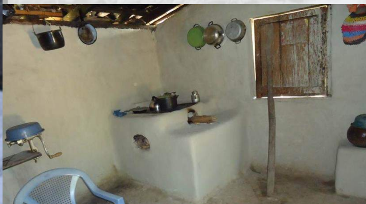
Inside kitchen walls and stove plastered and neatly organized / Paredes interiores de la cocina revocadas y bien organizadas
